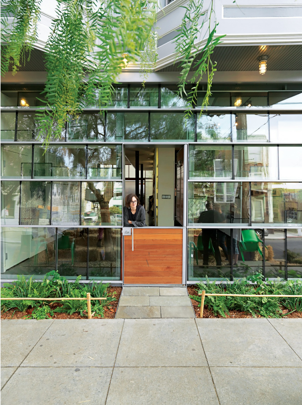
Dunbar and Astrakhan's low-cost, high-impact tour de force is a storefront facade constructed from salvaged double-insulated window glass panels arranged in a shingle pattern. Image courtesy of Justin Fantl Photography.
