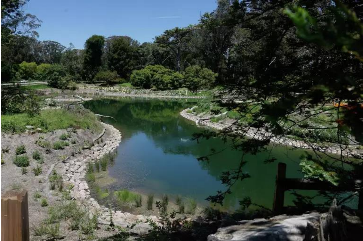
Golden Gate Park's Middle Lake, which has been dried up for decades, is now 7-feet deep with a clay bottom after undergoing a rehabilitation project. Lea Suzuki/The Chronicle
